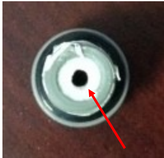
Undersink Top Spout Adapter Showing mineral buildup (Front View)
