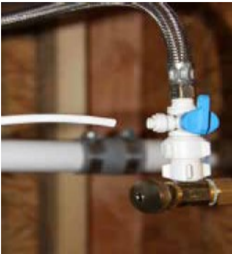
Angle Stop Adapter or T Valve installed at source water.
